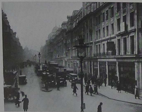
Regent Street, looking north from the Quadrant
